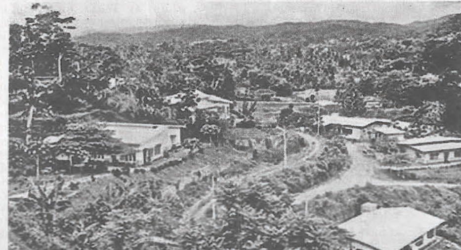
Watapuluwa Housing Scheme under construction
