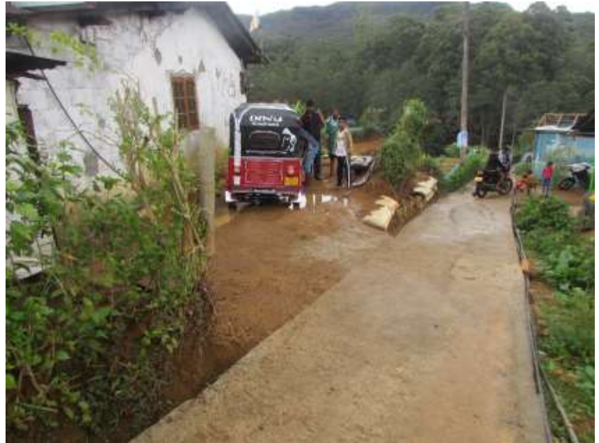
The completed internal access road in Kikilyamana GN division.
