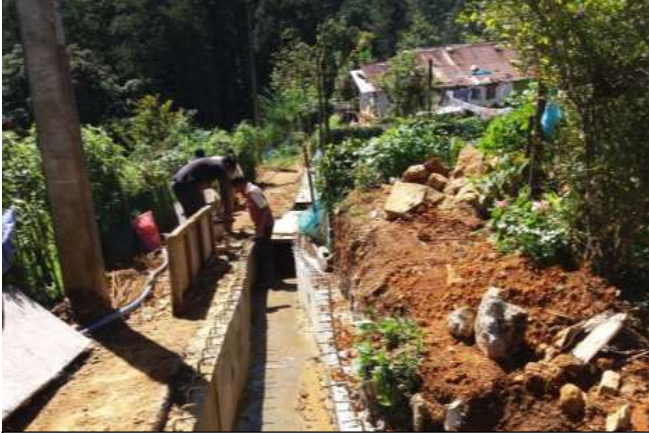
The internal road during construction.
