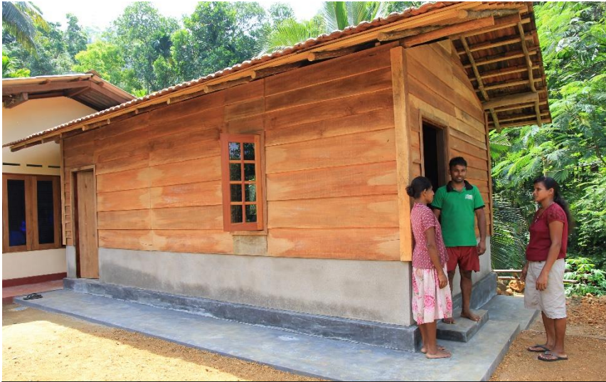
Newly constructed transitional shelter belonging to Sunil and Niroshini.
