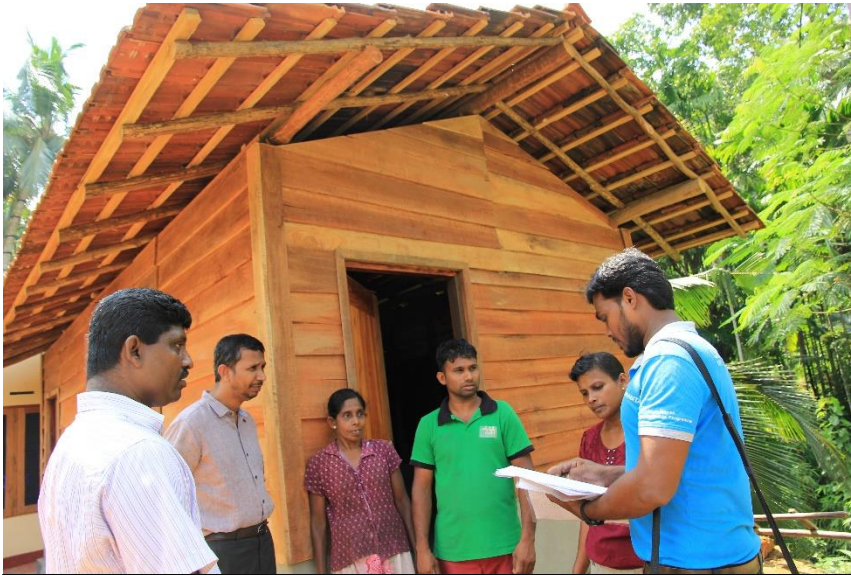
UN-Habitat technical team discussing the transitional shelter construction progress with Sunil Jayawansha's family.
