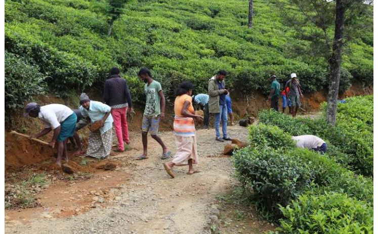
Community members clearing the roadsides through a 'shramadana' activity.
