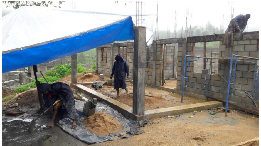
The CDC is currently under construction in Dunsinane estate, Nuwara Eliya.
