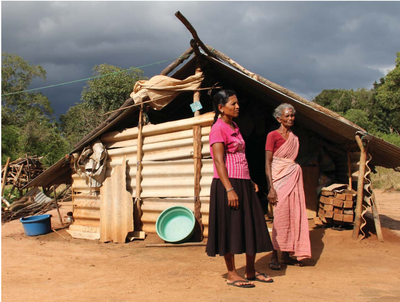
The harsh reality of temporary shelter: makeshift shelters made of cadjan, tin sheets and tent material formed the temporary homes of returnee families. Families lived in these shelters for months, until permanent houses were built. © UN-Habitat / Nipuna Kumbalathara
