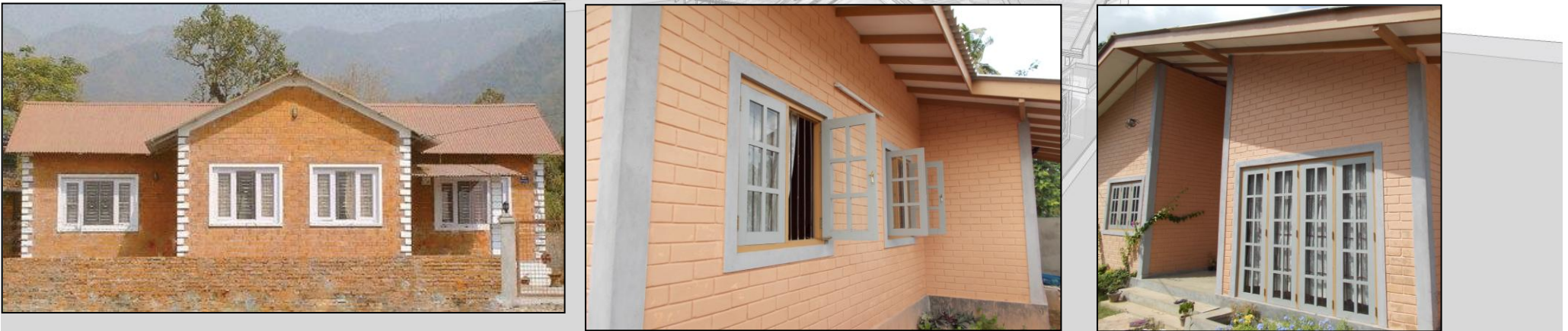
Un-plastered walls with plaster bands (architraves) along edges
