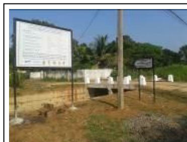
The built culvert and drainage wall ensuring access on traditional routes
