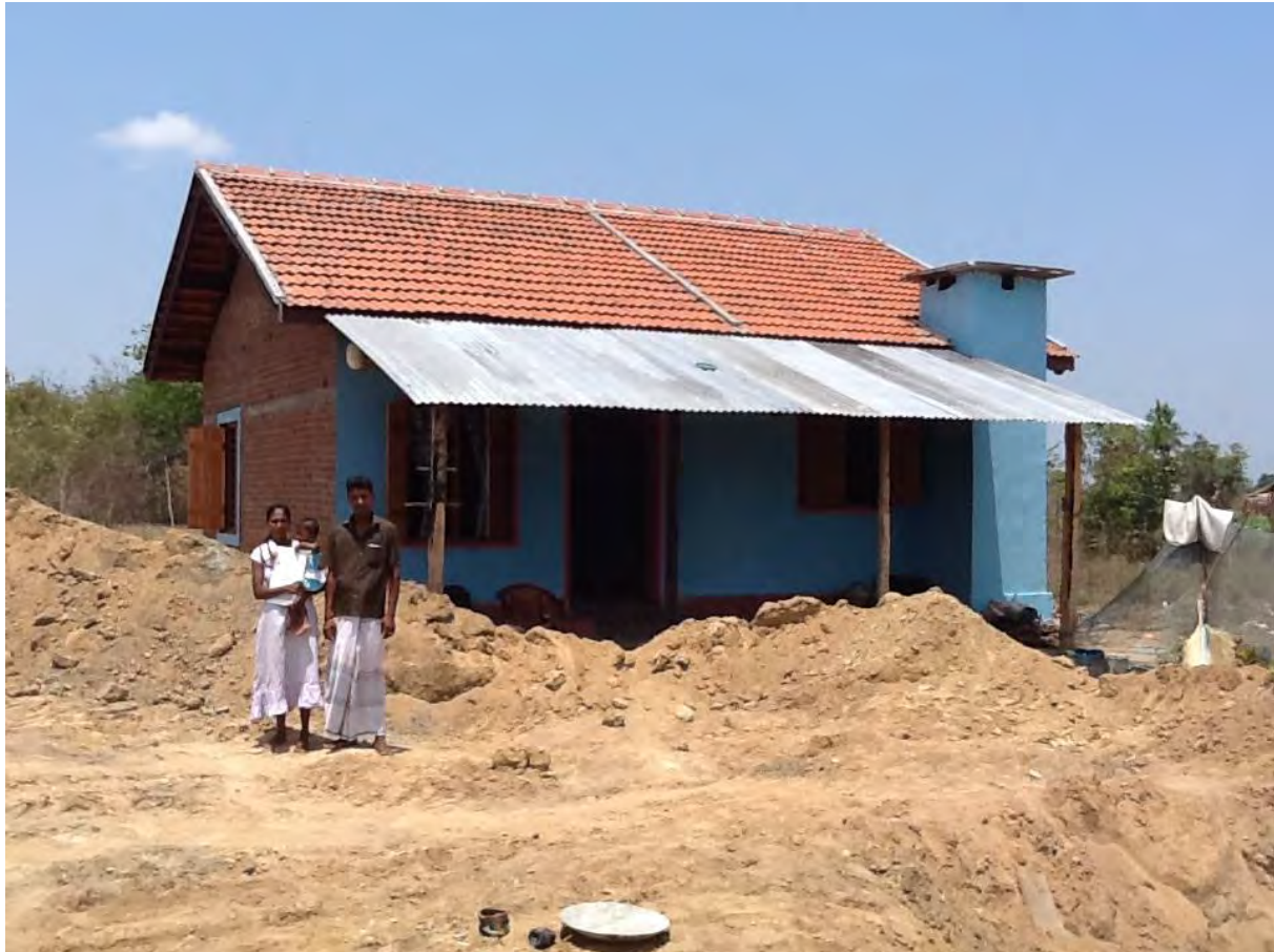
Illustration 11: Observation no. 27 (Veppavedduwan village): only one strip per eave insufficient to safeguard roof from strong winds (Source: Mario Martelli, September 2014)
