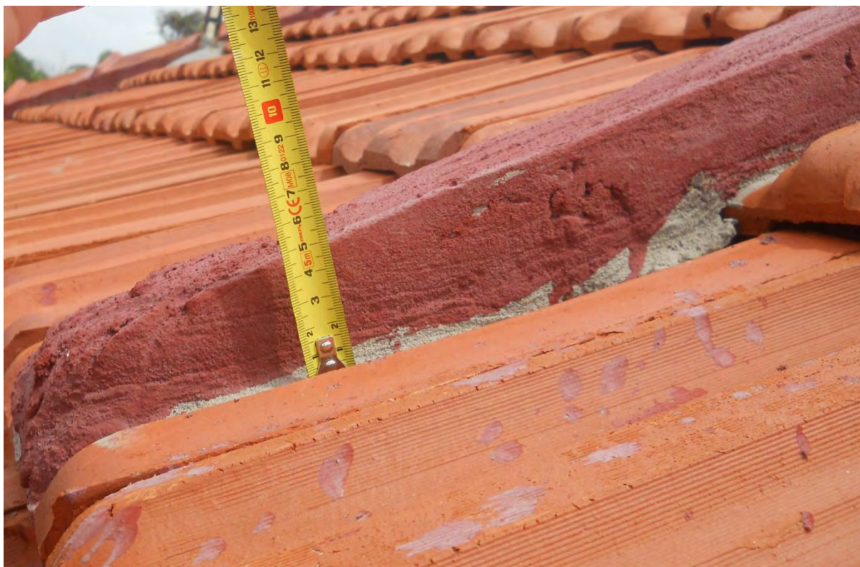
Illustration 12: Observation no. 13 SDC (Kilali village): typical strip dimensions: due to the absence of metal reinforcement, they appear insufficient to resist cracking, likely due to roof and tiles settling (Source: Mario Martelli, September 2014)
