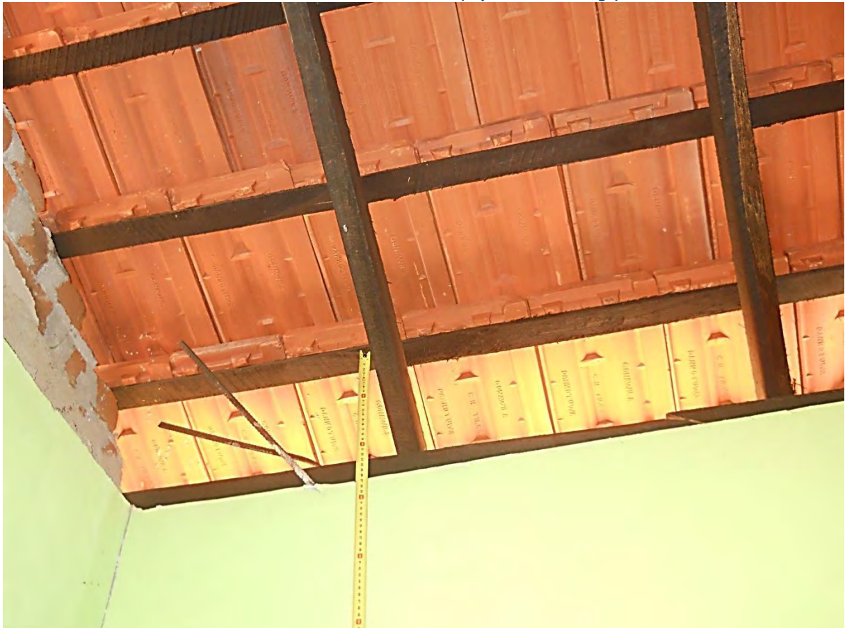
Illustration 9: Observation no. 27 (Veppavedduwan village): rafter spacing (and reinforcement bars not appropriately bent) (Source: Mario Martelli, September 2014)
