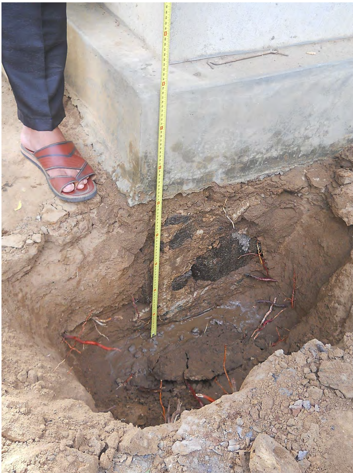
Illustration 10: Observation no. 9 (Piramanthanaru village): foundation check gave a good result and confirmed the appropriate implementation of this important structural component (Source: Mario Martelli, September 2014)
