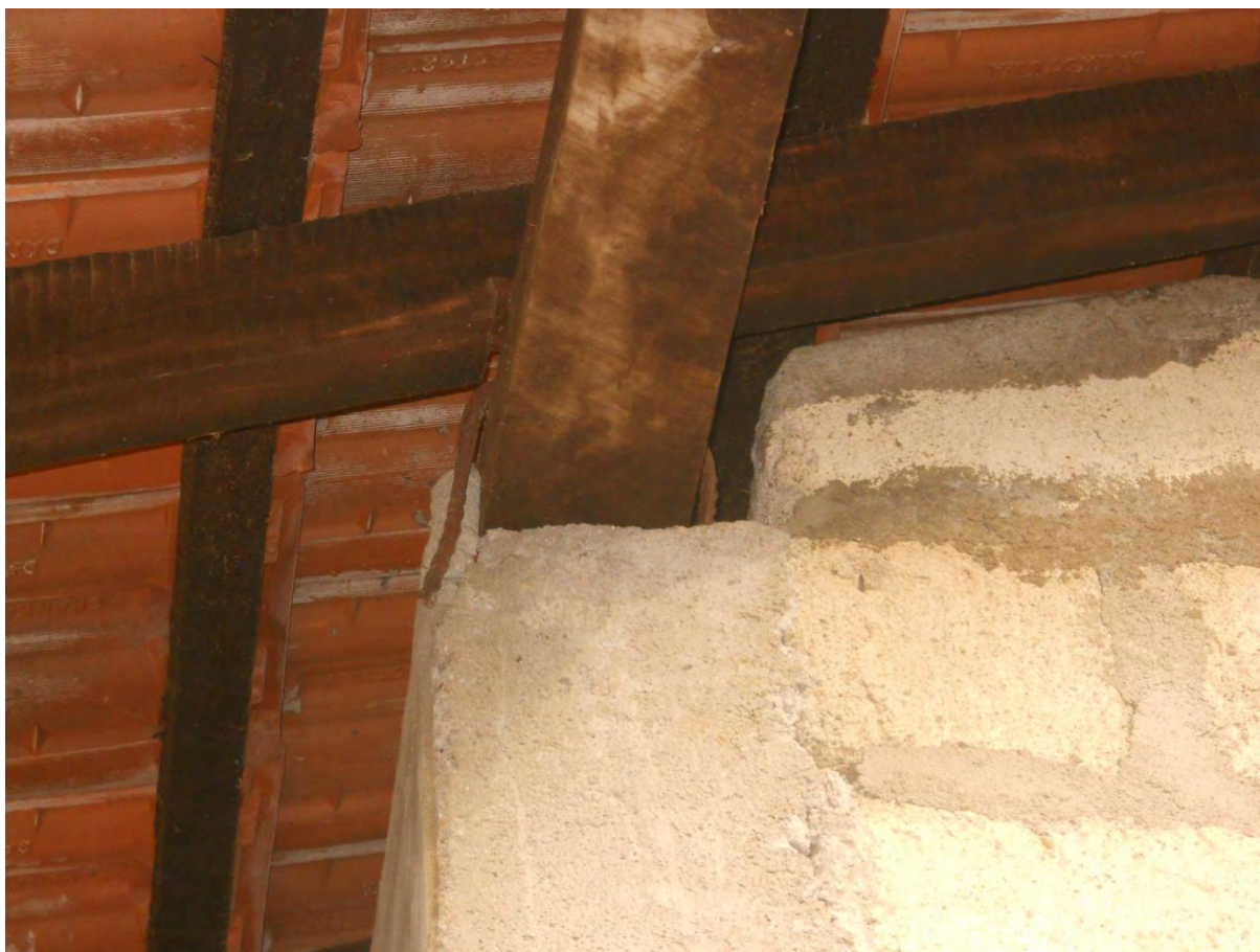
Illustration 15: Observation no. 11 (Piramanthanaru village); detail: corner column, reinforcement bars and wall plate (Source: Mario Martelli, September 2014)
