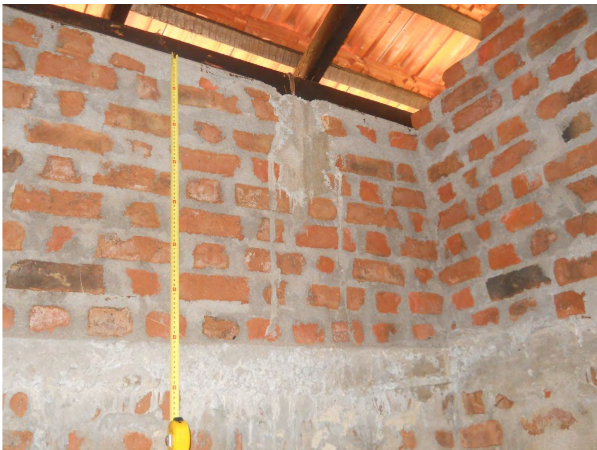
Illustration 6: Observation 25 (Veppavedduwan village): structurally unsafe fake column (Source: Mario Martelli, September 2014)
