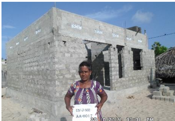
House construction in progress at wall plate level.
