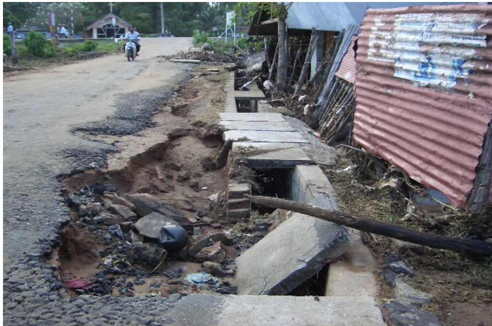
DAMAGE OF STORM WATER DRAIN IN DUTCHBAR
