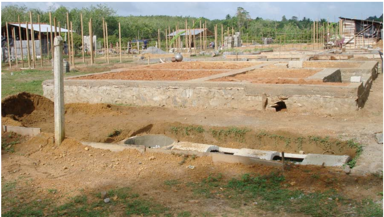
Houses being constructed at Raigamwatta
