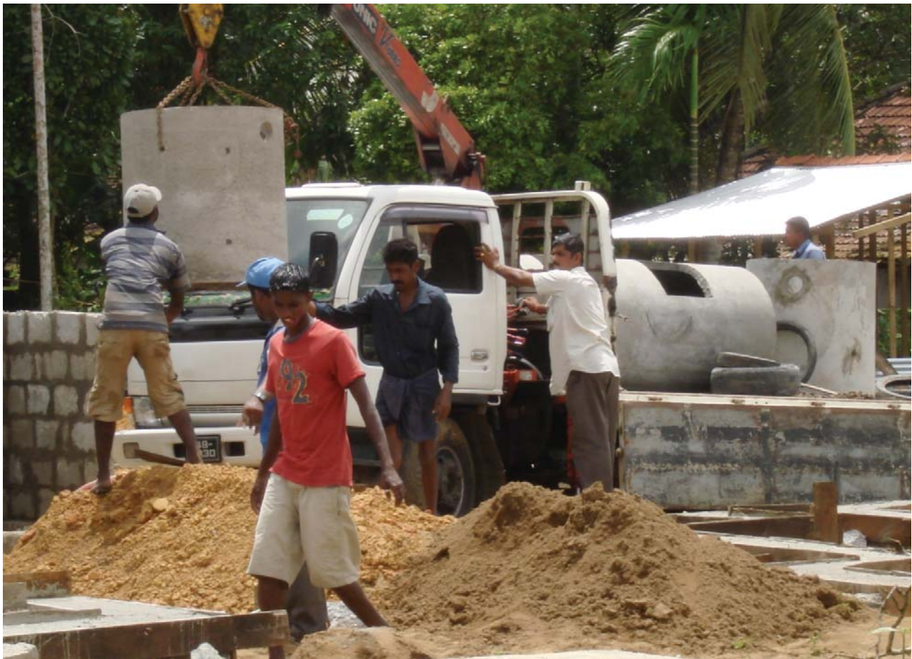
Transporting septic tanks to the site
