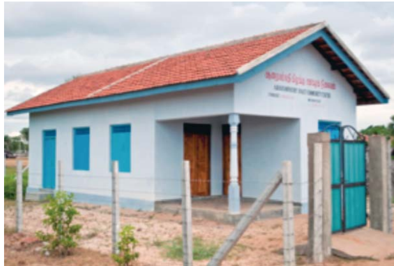
Community centre constructed under the CRRP Project
