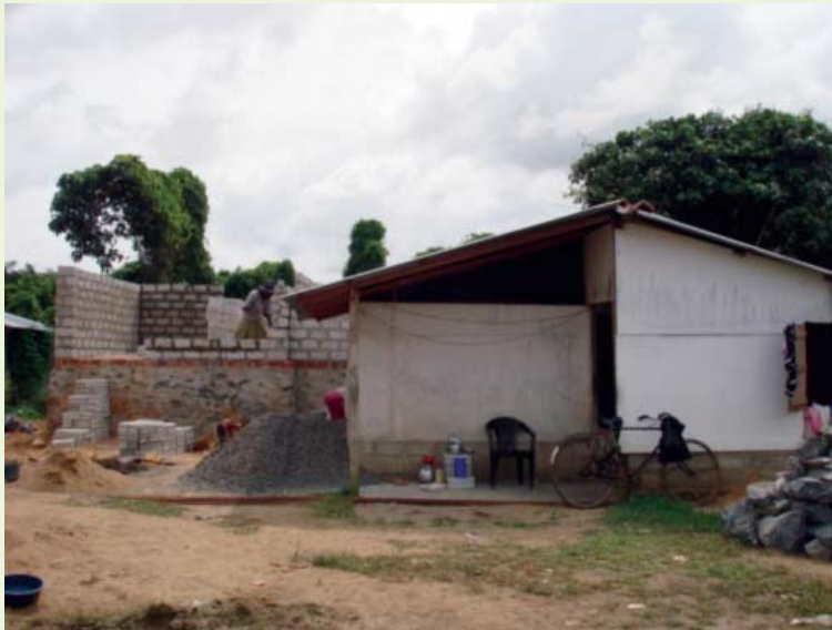
Construction of raised plinth levels.
