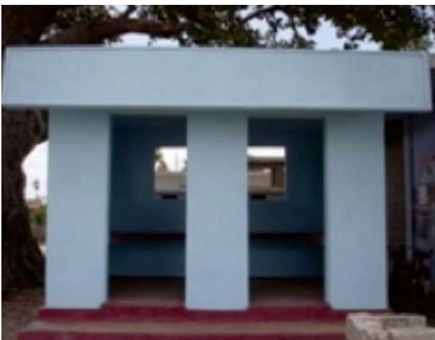
Bus Halt constructed in Ampara
