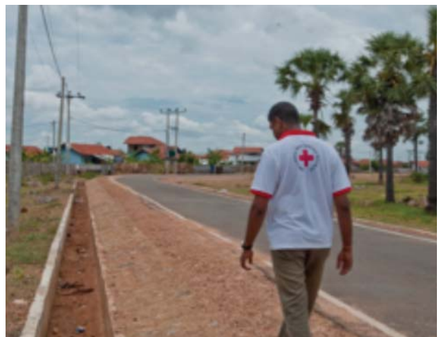
An access road constructed in the Jaffna District
