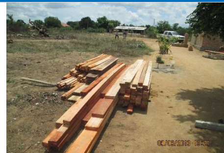
Timber: Before treatment
