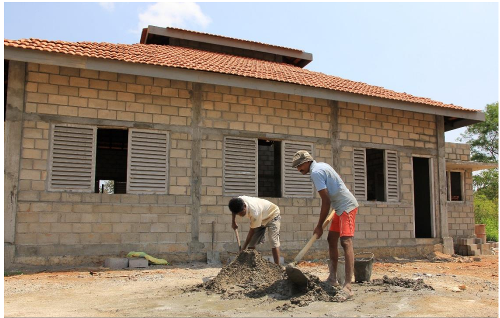
New Sivanagar preschool under construction.
