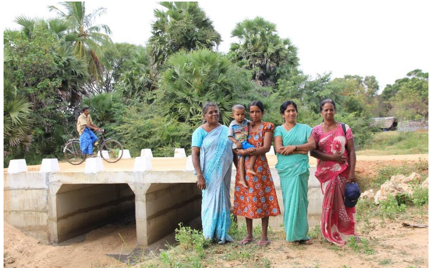
Puliampokkanai WRDS members near the newly constructed storm water drainage system.
