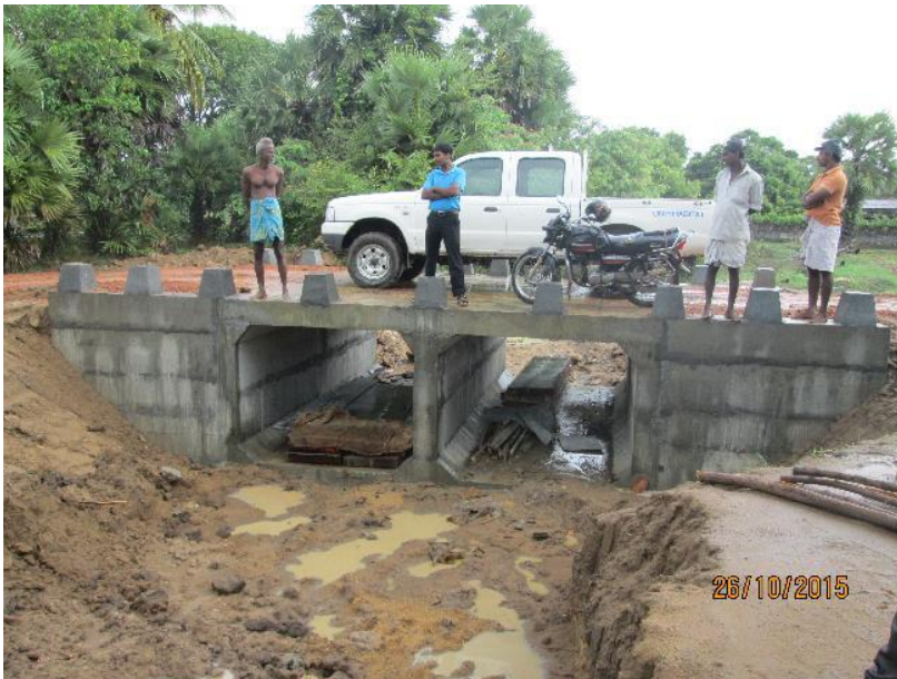
UN-Habitat technical team monitoring the construction progress with community members.
