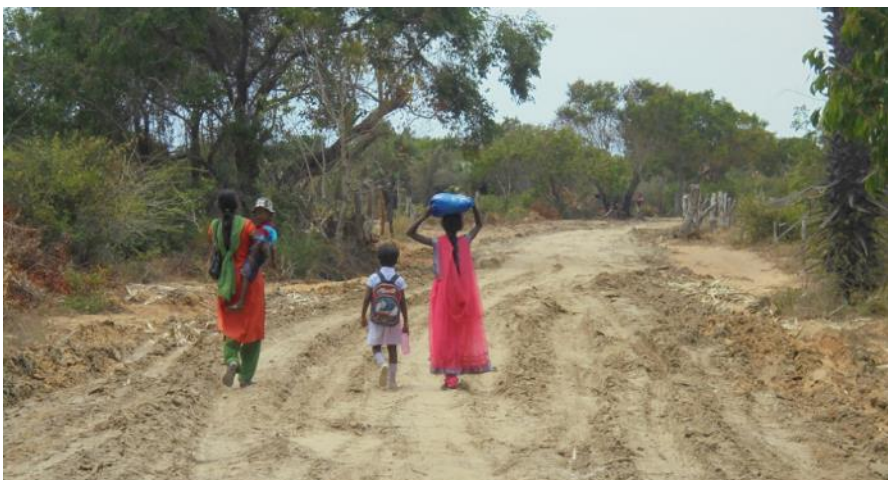
The internal access road, before repair.
