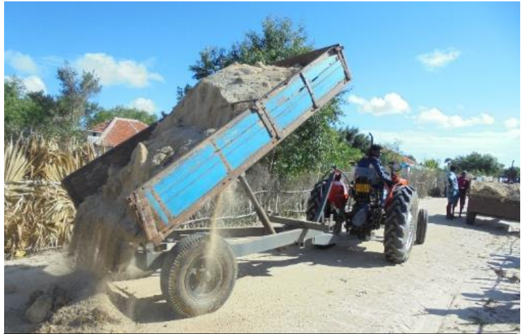
The road under construction.
