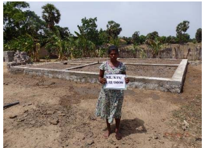
The house at foundation level.
