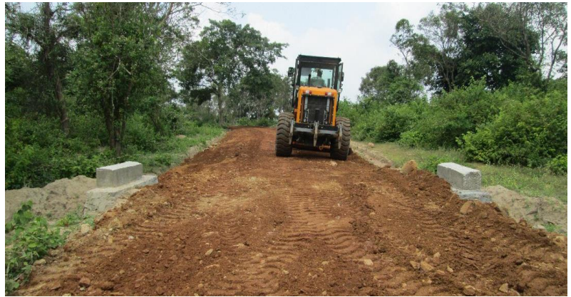
Road rehabilitation work in progress in Karaveddy village.
