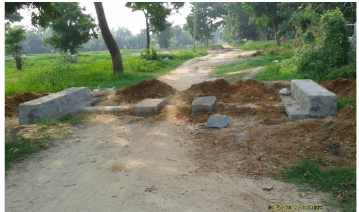
Culvert under construction on the cemetery road, Karaveddy.
